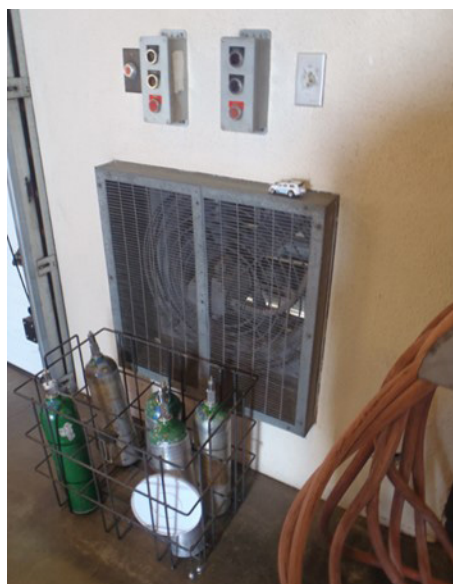
Figure 2. Five small compressed gas cylinders partially blocking the intake of a floor level wall exhaust fan at Station 17. Photo by NIOSH.
